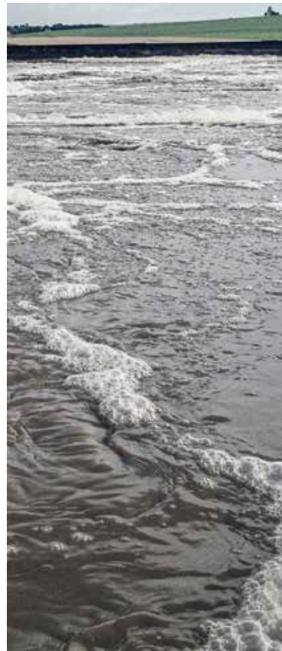
Seven-path ejectors in a 2 200 m 3 aeration tank in the cooking oil industry in Brazil
