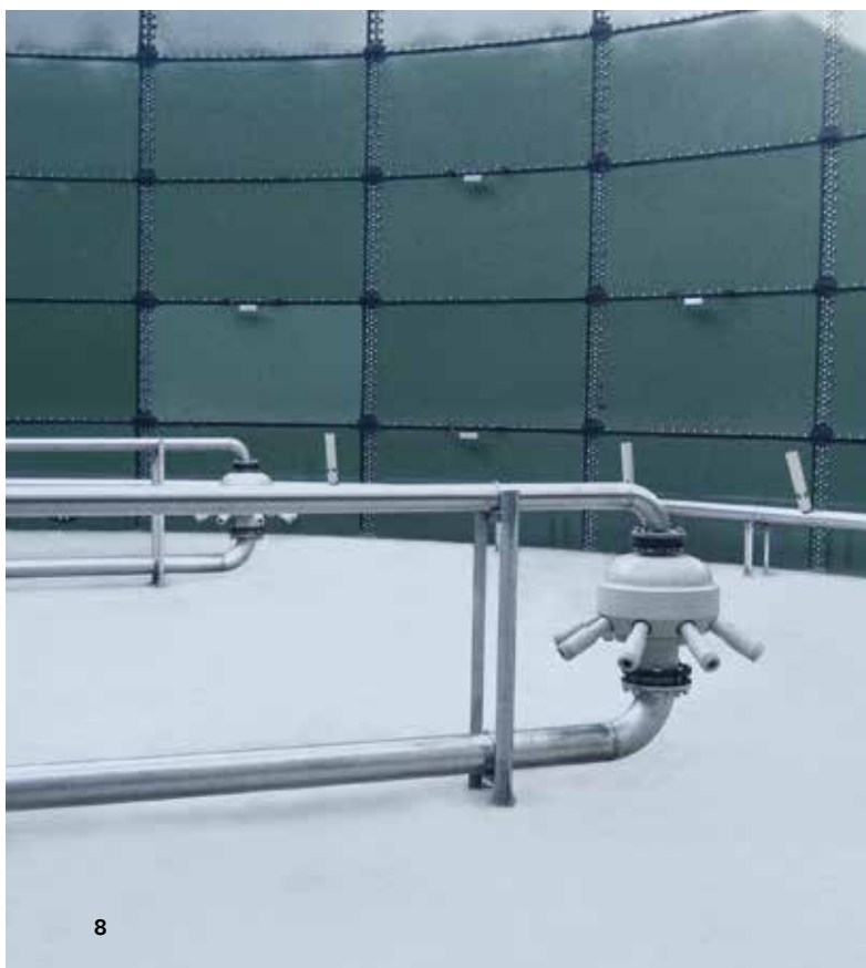
Ejectors and mixing nozzles for aeration and complete intermixing in an SBR reactor
