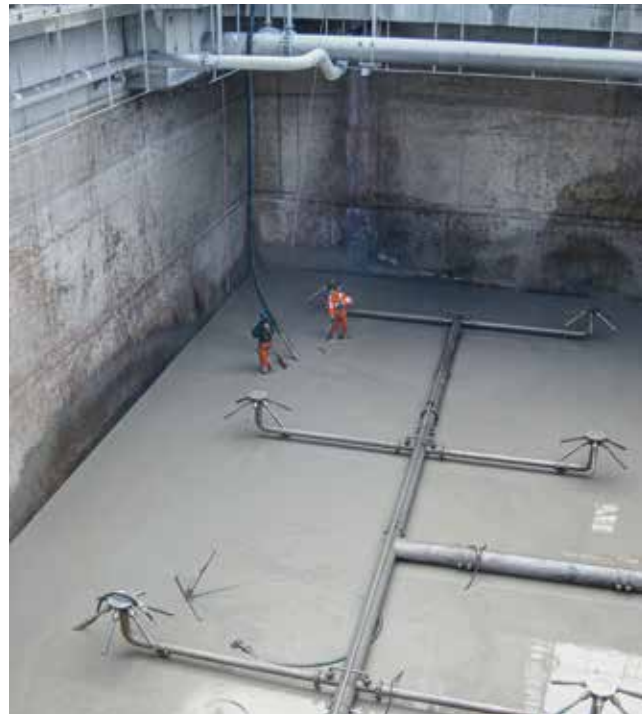
Oxygen transfer system in the aeration tank of the Gebr. Lang GmbH paper mill in Ettringen, Germany. The six-path ejectors are supplied with gaseous oxygen from a stationary tank system.
