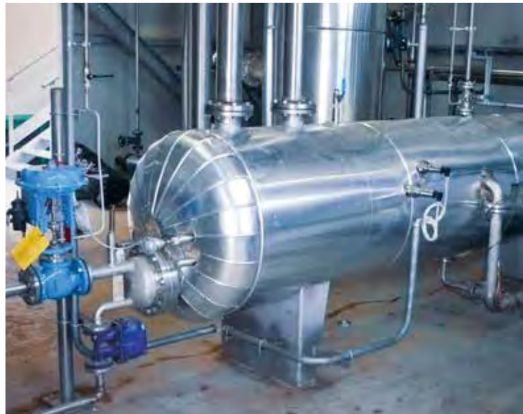
A Körting ICE Condensation Vacuum System's melting vessel
