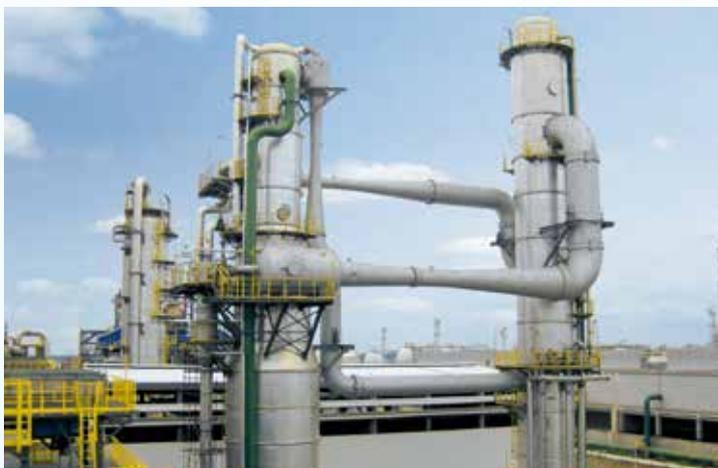
24 MW steam jet chilling plant Petro China/Sichuan refinery, cooling of 2 300 m<sup>3</sup>/h from 29 °C to 20 °C
