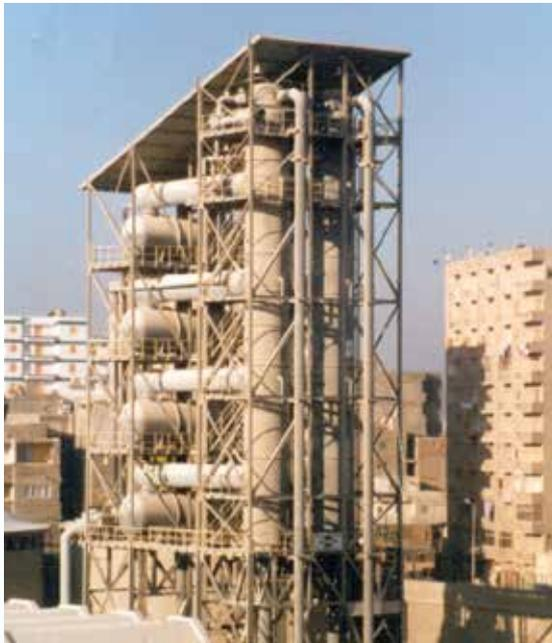
28 MW steam jet chilling plant in Egypt, cooling of 1 600 m<sup>3</sup>/h from 35 °C to 20 °C
