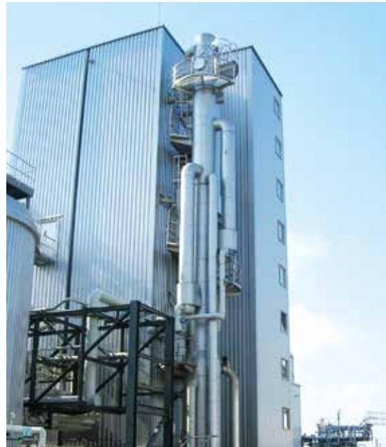
About 1.4 MW steam jet chilling plant in Stendal, cooling of about 72 m<sup>3</sup>/h from 25 °C to 8 °C
