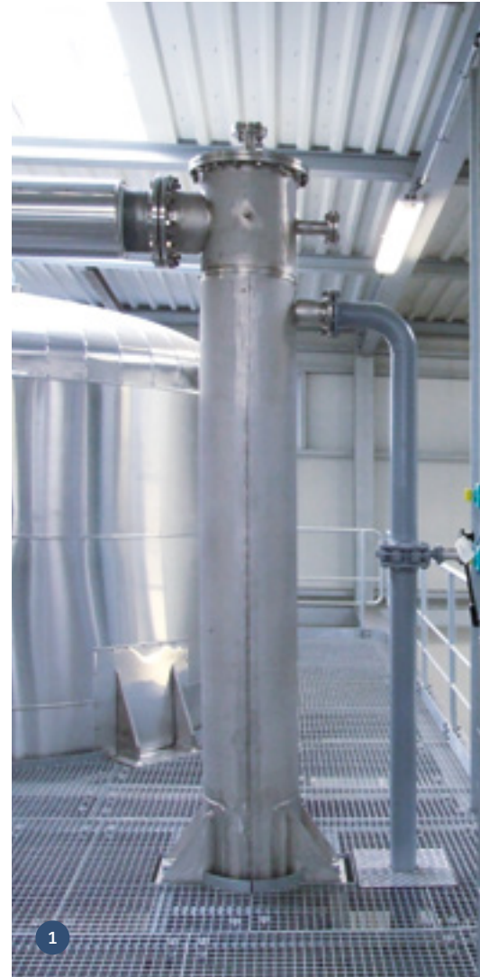
1/2) Vacuum system with indirect condensation
