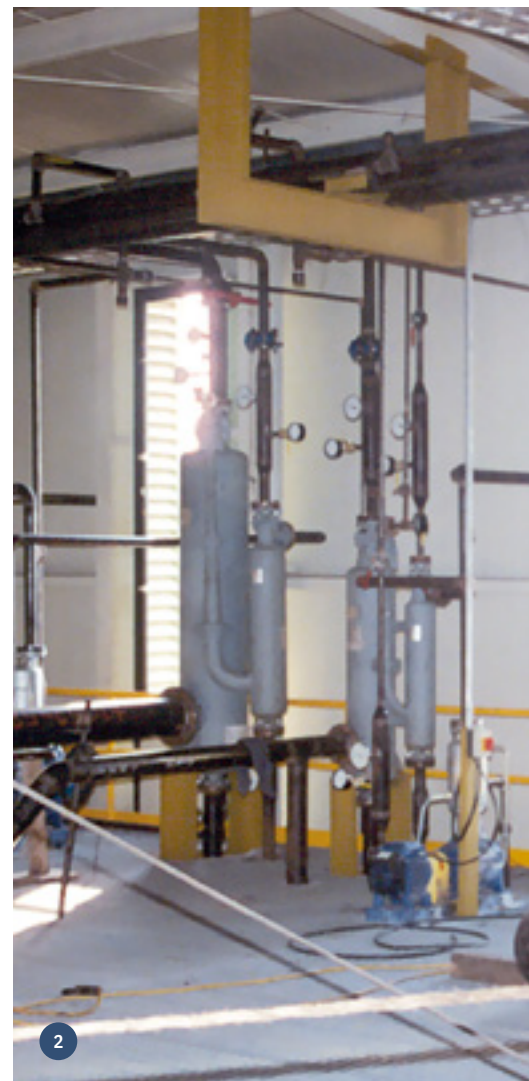
1/2) Conventional vacuum systems operating with mixing condensers
